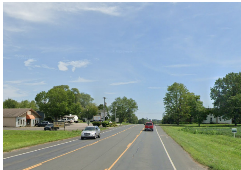
Streets within Dorr, Moline, and developed subdivisions are generally paved.
